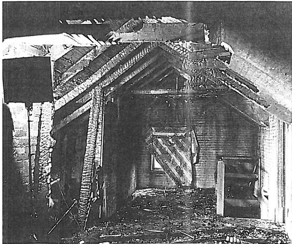
CENTER ROOM OF ATTIC
