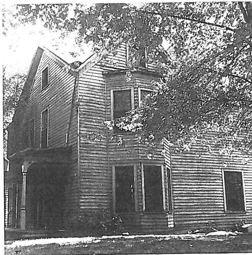
REAR AND WEST SIDE OF DWELLING
