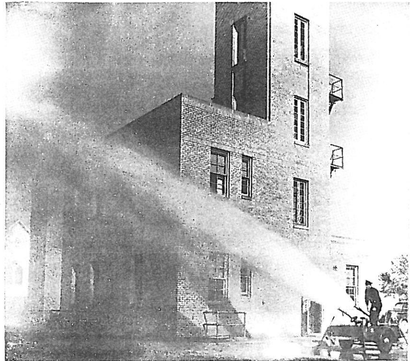
Showing Reach of Fog Cones
