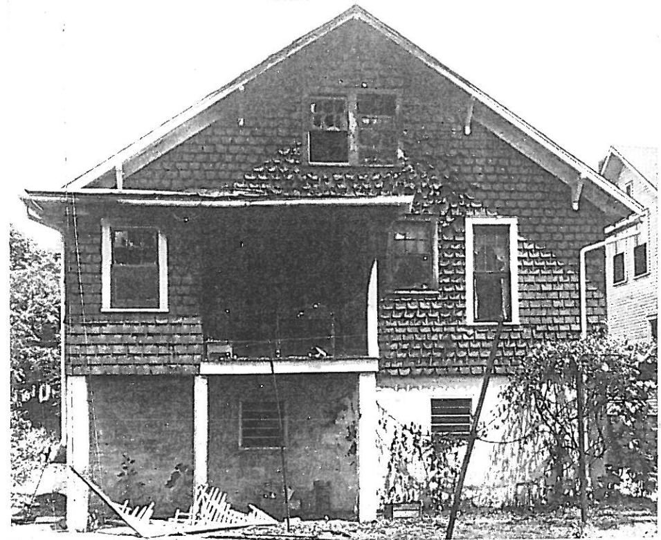
REAR VIEW OF DWELLING
