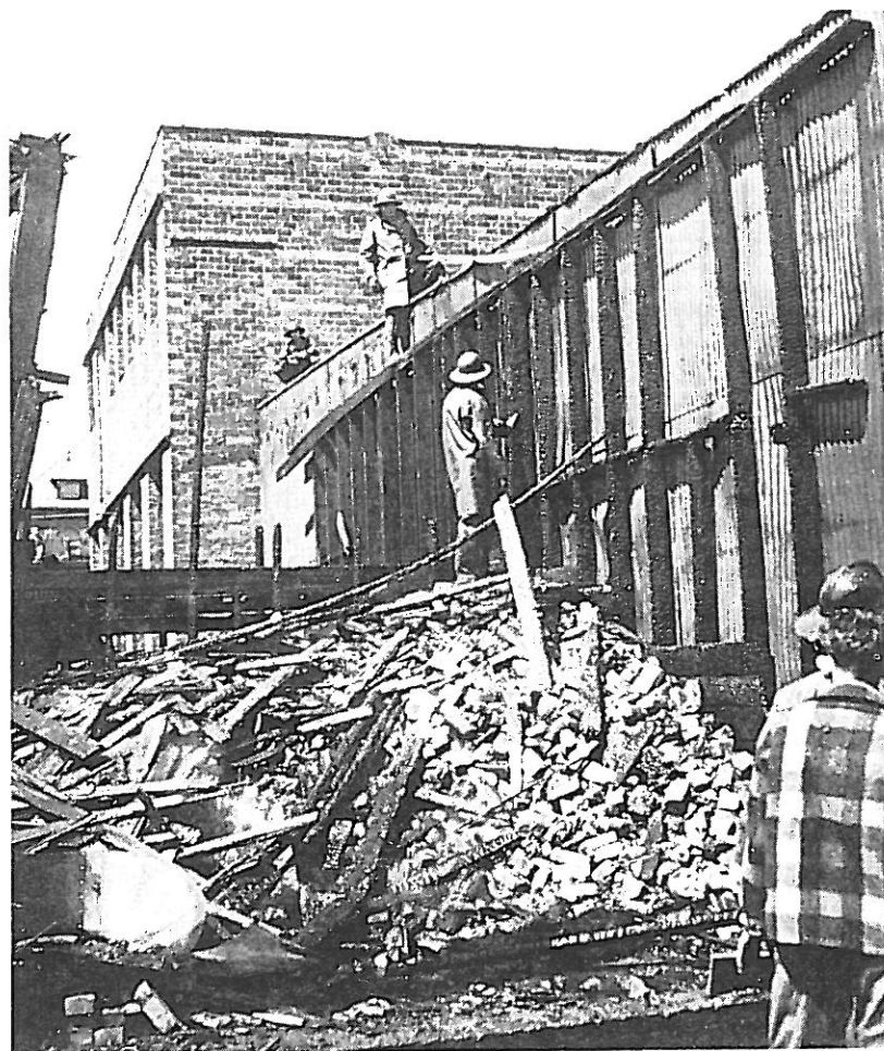
REAR VIEW OF WAREHOUSE Shows where fire originated.
