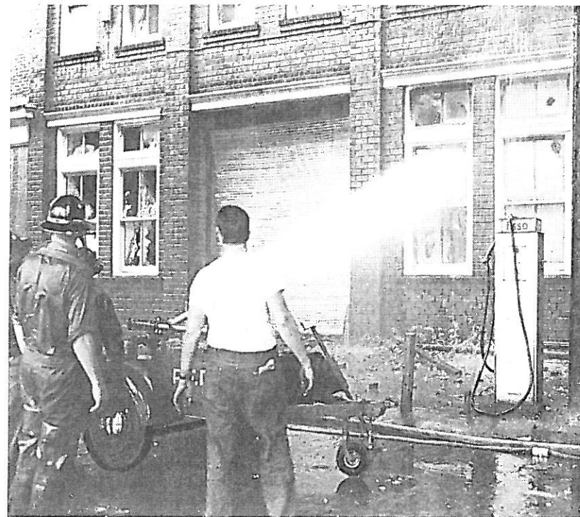
C-6. Fog cone from monitor unit being directed into 113 Ann Street Parkersburg, W. Va.
